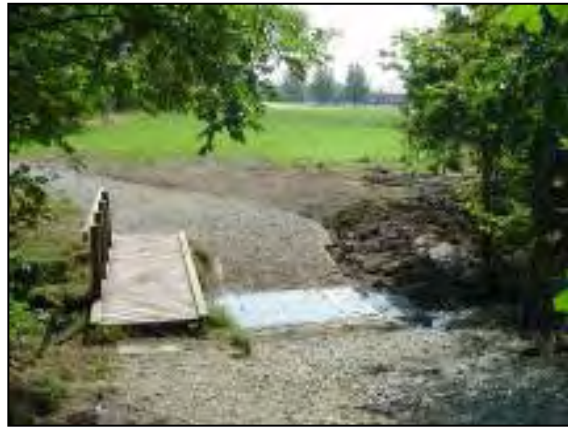
Plate: 50 Location: Chesham Characteristic: Ford over brook
