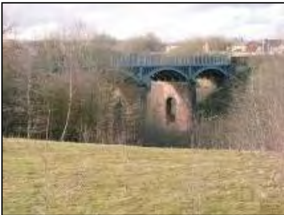
Plate: 81 Location: Prestwich Characteristic: View of old railway bridge
