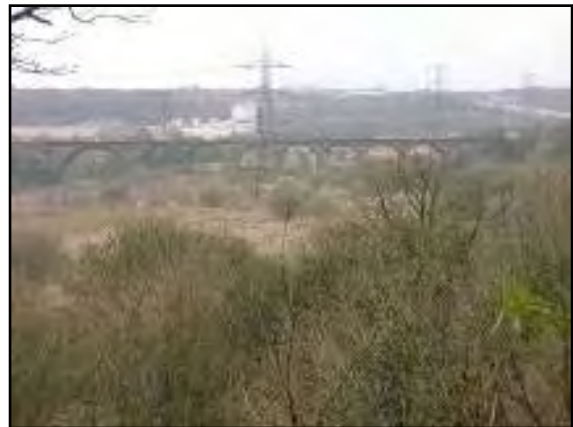
Plate: 76 Location: Irwell Characteristic: Clifton Viaduct
