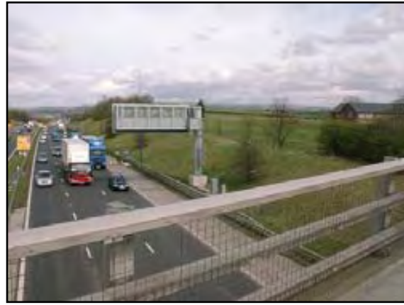
Plate: 38 Location: Bridge near Unsworth Characteristic: M66 motorway bridge
